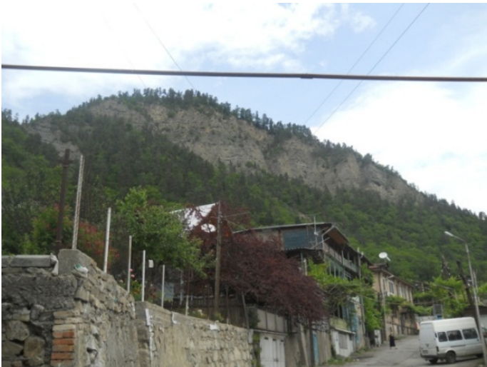
Figure 6. City Borjomi, rockfall area.
