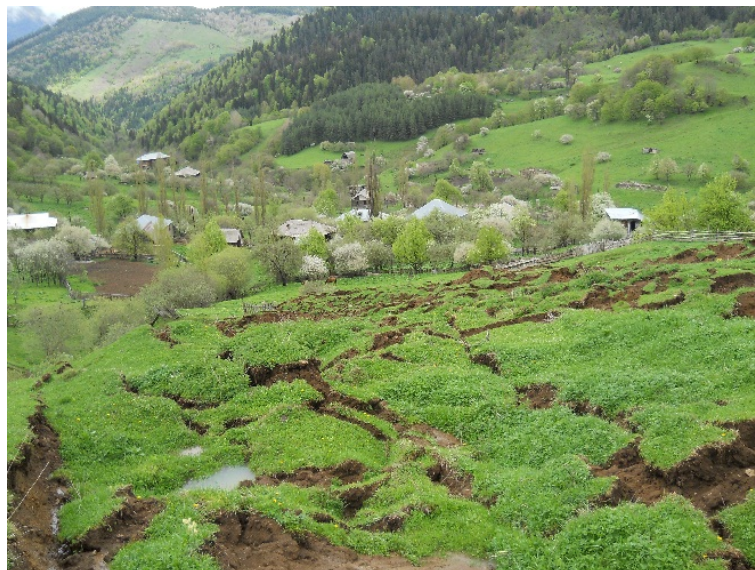
Figure 11. Village Didi Mitarbi landslide.
