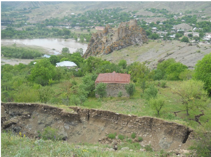
Figure 15. Village Gaghma-Atskuri landslide.
